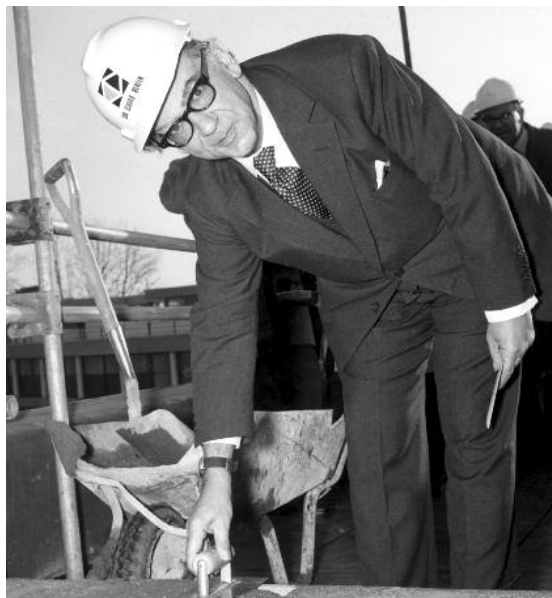
Figure 2. Isaiah Berlin 'topping out' the new Wolfson College buildings, December 1972. Photo: Shepherd Building Group Ltd.
