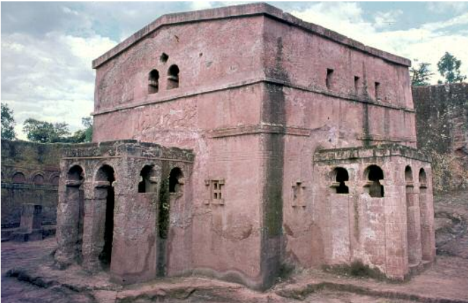
Figure 6. Beta Maryam (the church of St Mary) is one of the most elaborate of the Lalibela hypogea. Carved from bedrock (a volcanic tuff), it rises 10 metres from the floor of a large sub-rectangular court. Internally, it follows a basilican plan and bears fine carved and painted decoration.
