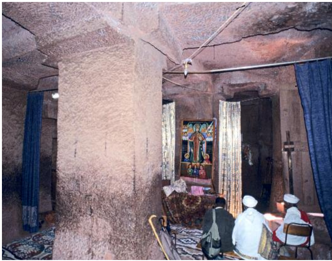
Figure 5. Beta Gabriel (the church of the Archangel Gabriel) is one of the oldest hypogea at Lalibela. Several phases of modification may be recognised. Initially defensive, its subsequent conversion to ecclesiastical use involved the excavation of an additional chamber (reached through the curtained doorway seen behind the priests in this photograph) to serve as the sanctuary. At about the same time the previously flat ceiling was re-carved to represent capitals and beams.
