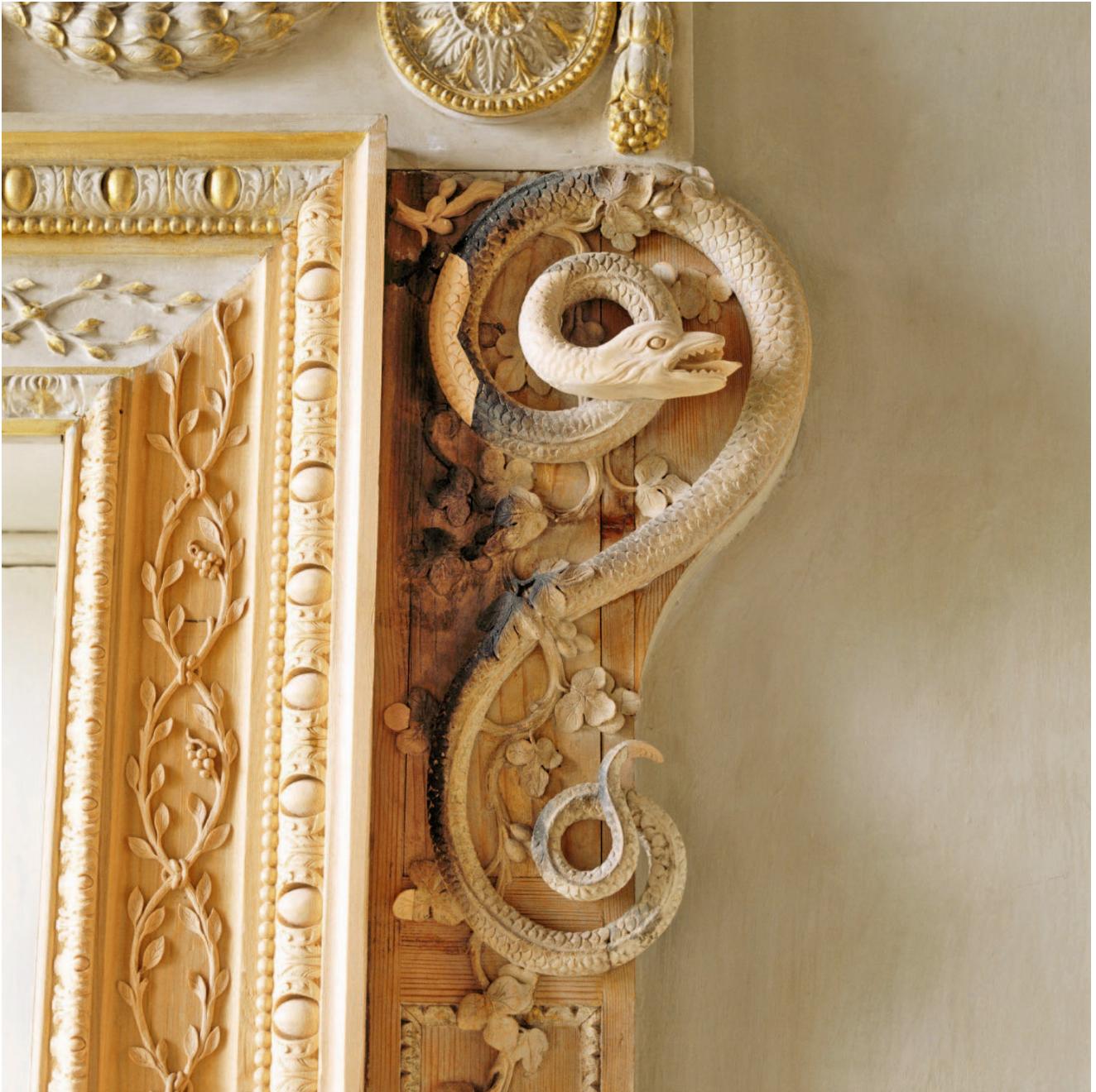
Figure 1. Conservation choices. After the fire at Uppark, the serpent 'capitals' of the Saloon doorcases were restored, but scorch marks were left on the woodwork. Photo: ©NTPL/Andreas von Einsiedel.
