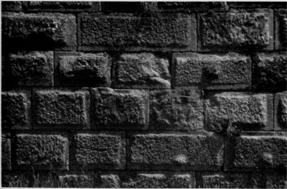
b. Terrace wall at Delphi
