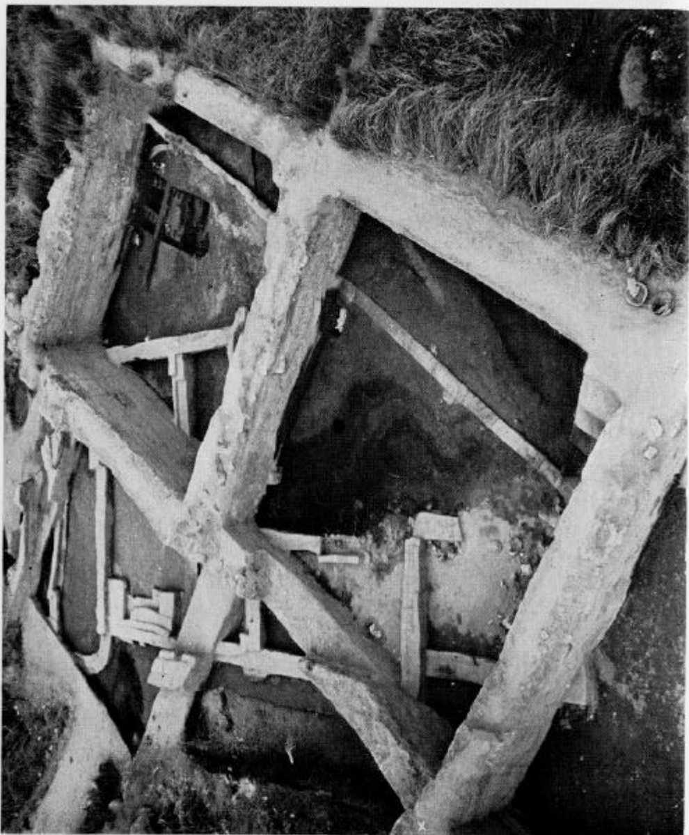
IV. Tell el-Dab'a, stratum G, building compound of the late 13th dynasty inhabited by Canaanites. Main building with two rooms and a tomb in front of the entrance. Two subsequently attached rooms with numerous amphorae
