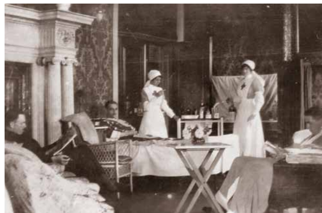
Figure 3 Ward in the Dining Room on the Ground Floor.
