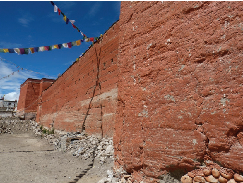
Figure 8. View of the rammed earth wall surrounding the city of Lo Manthang in Mustang, Nepal. (Image: Durham UNESCO Chair).
