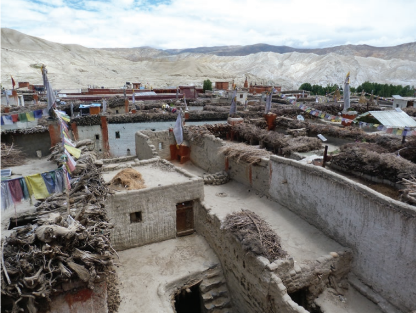
Figure 7. View of the flat mud roofs in upper Mustang, Nepal (Image: Durham UNESCO Chair).
