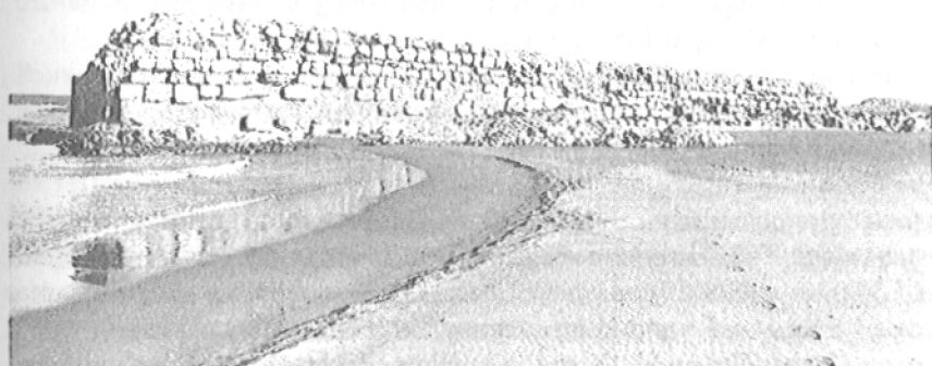
Figure 5. View of the Empúries breakwater from the west.
