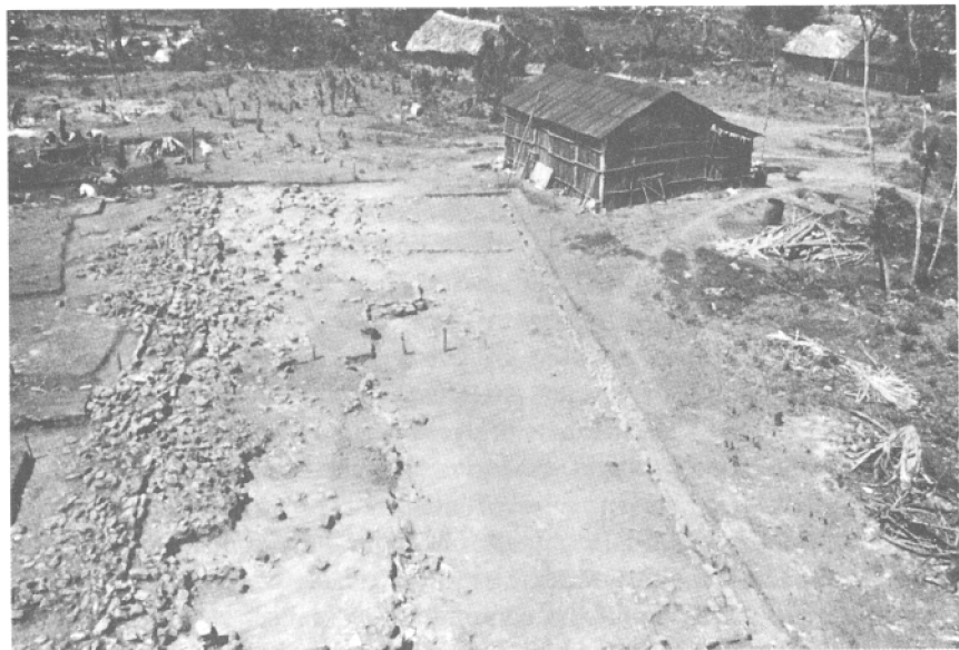
Figure 2 Structure N11-18, Lamanai. The building, 22 metres long, was probably the cacique's residence.
